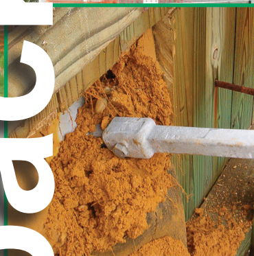
Typical installation of helical tieback anchors to support walls during excavation.
