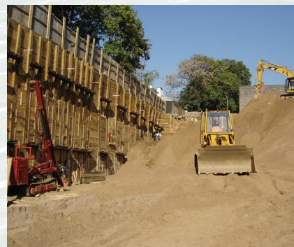
Typical installation of helical tieback anchors to support walls during excavation.
