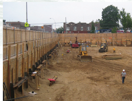
Typical installation of helical tieback anchors to support walls during excavation.
