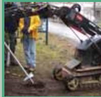
Shoring system attached to square helical piles
