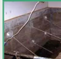
Twenty-four tiebacks installed to support bowing wall
