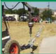
MacLean-Dixie foundation systems install quickly and easily. They're simply screwed down into stable soil strata using hydraulic torque motor installation equipment. There's no excavating or spoils to remove. No hammering or vibration that can disturb surrounding structures.
