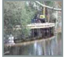
Concrete pile caps cast to support timber columns
