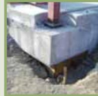
Building load directly on installed square helical piles
