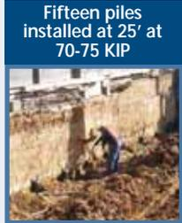
Fifteen piles installed at 25' at 70-75 KIP
