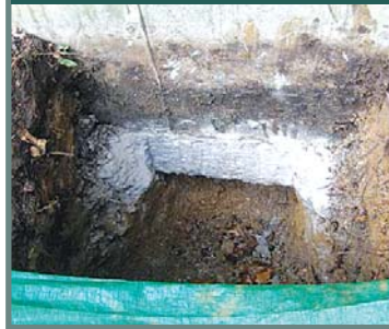
Excavated 3' x 4' hole to foundation base
