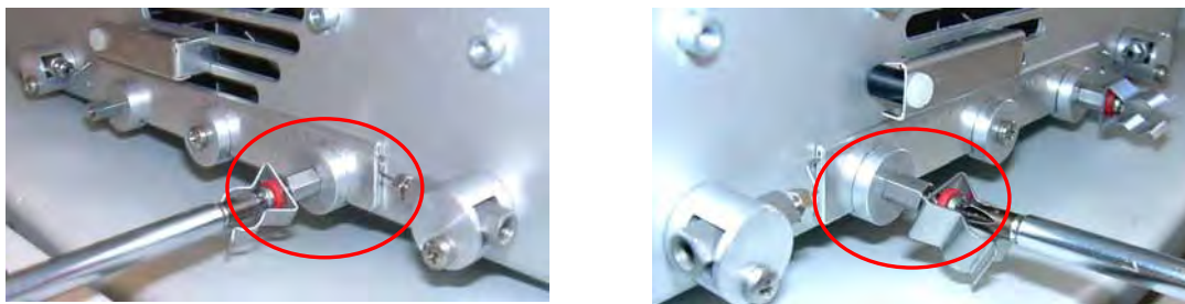
Fig. 21: Installing the column clips
