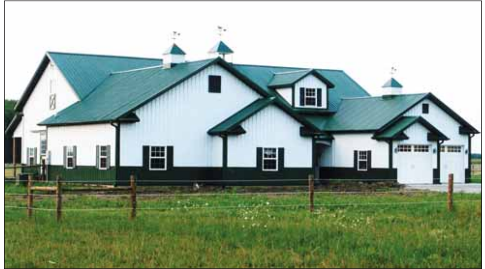
Figure 22. Although any exterior finish may be used, steel siding and roofing are popular due to economy and maintenance-free durability.
