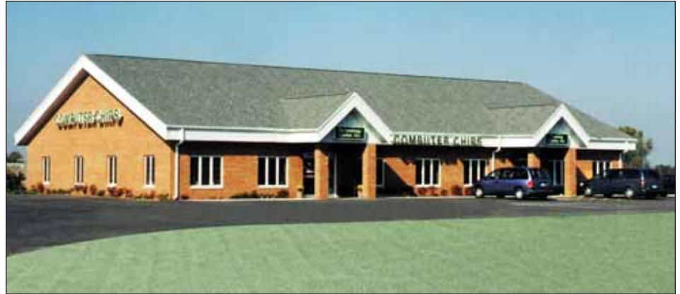
Figure 36. Many mistake this post-frame building for a less thermally-efficient brick building.
