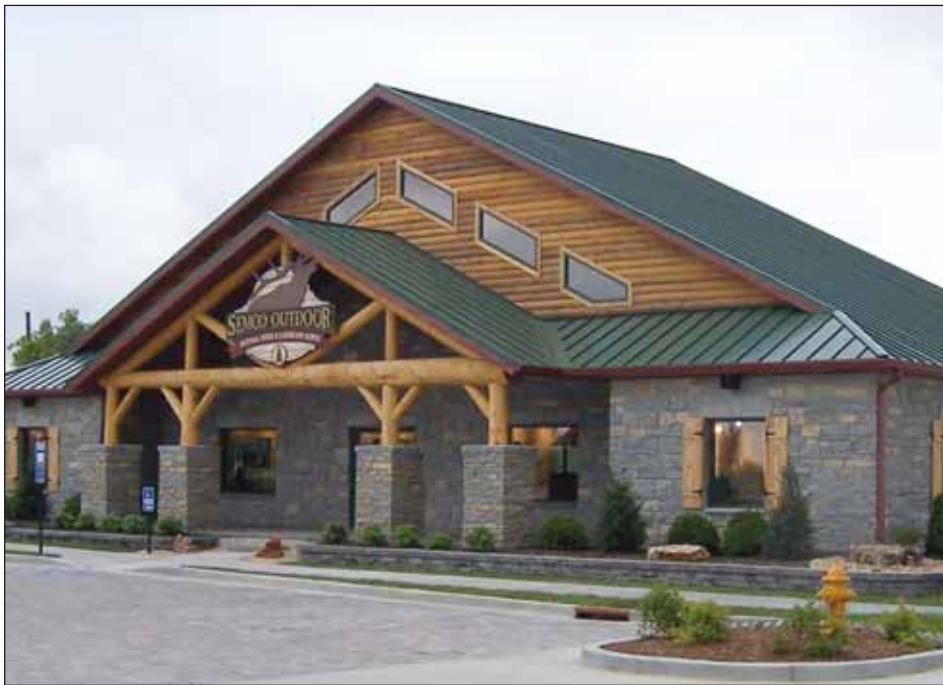
Figure 4. Post-frame building with stone and log facade.
