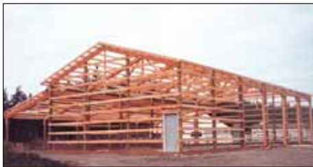
Figure 11. A typical post-frame building frame.
