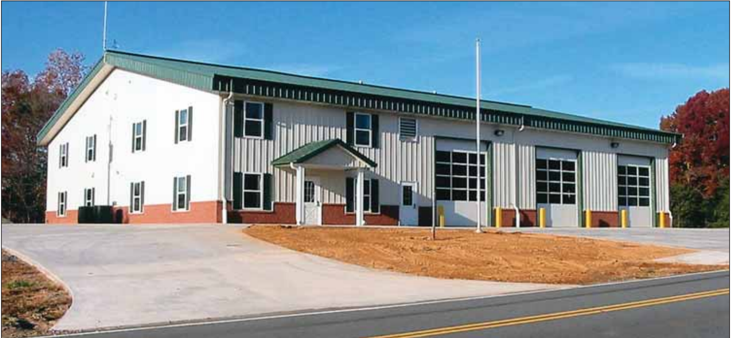
Figure 21. Post-frame allows high sidewalls and wide clear spans for mixed uses.
