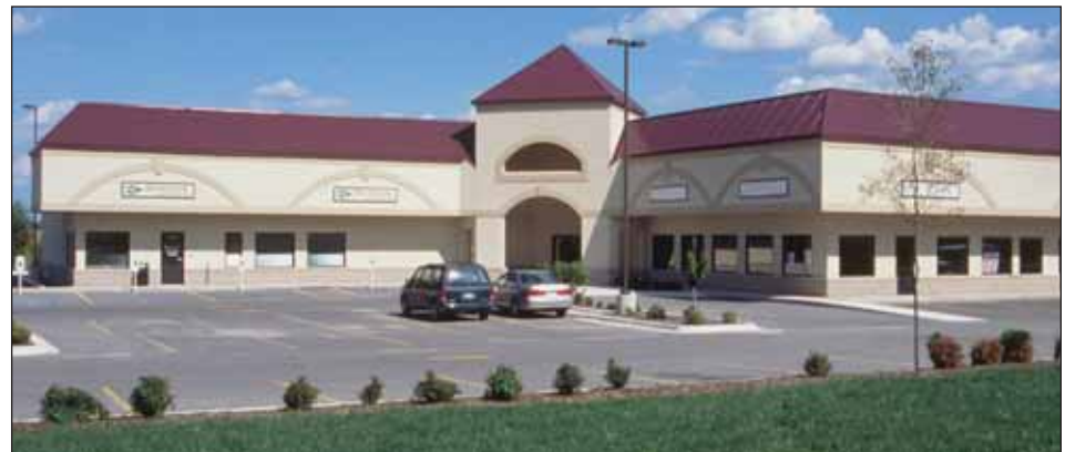
Figure 20. Post-frame is an excellent choice for strip malls and other retail buildings.
