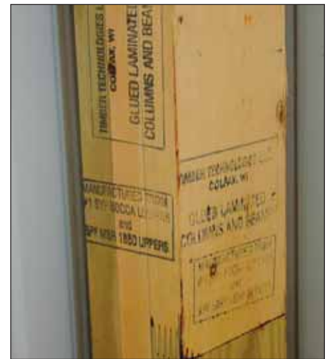
Figure 9. Finger-jointed glue-laminated columns provide one of several good post options. Note treated wood spliced to the bottom end.
