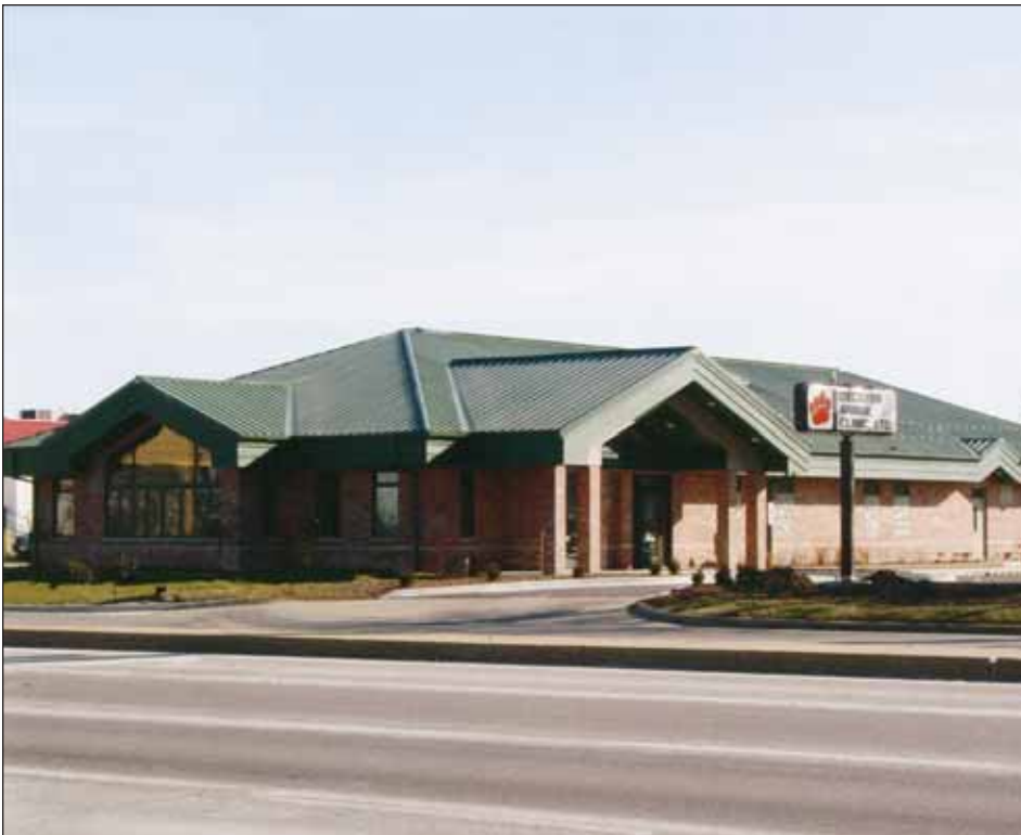
Figure 8. Mortarless brick and stone siding products allow design professionals new opportunities to create much more economical and energy-efficient buildings using post-frame techniques.
