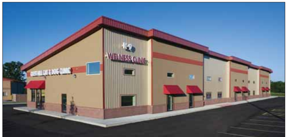
Figure 37. A post-frame veterinary facility.
