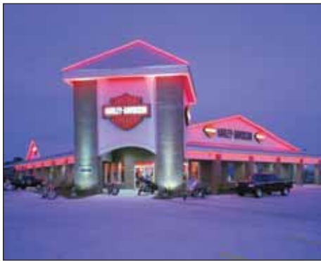
Figure 27. Post-frame retail facility with large interior clear-spans and ample room for show rooms and mechanic's shop.
