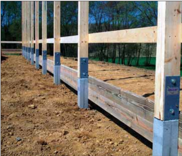
Figures 14 & 15. Pre-cast concrete piers provide one of several foundation options unique to post-frame.
