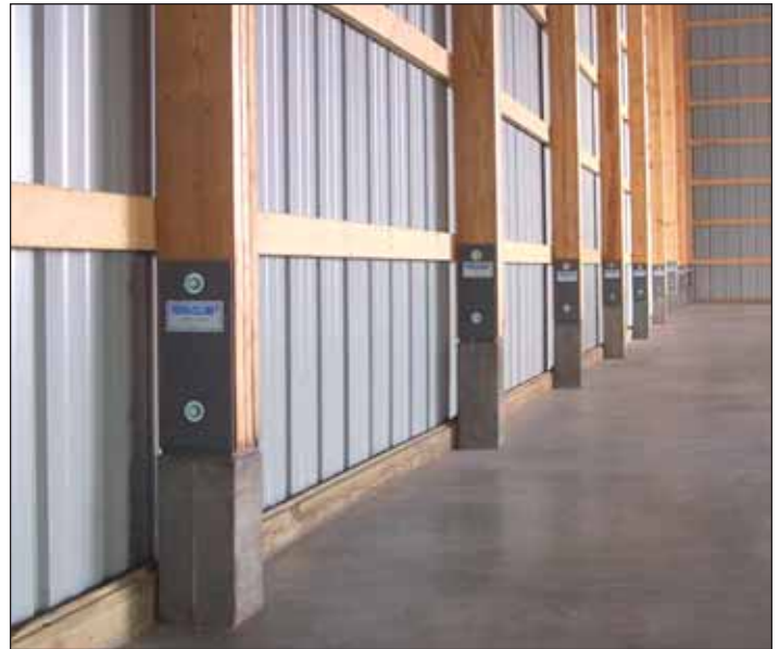
Figures 14 & 15. Pre-cast concrete piers provide one of several foundation options unique to post-frame.
