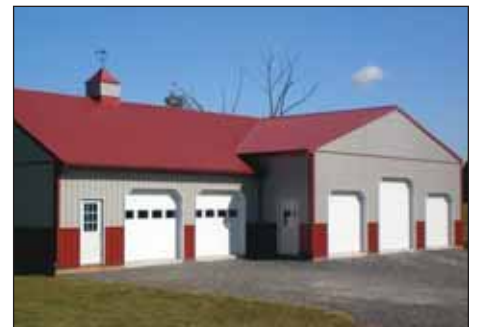
Figure 7. Post-frame is the most economical and versatile option for commercial and residential garages.
