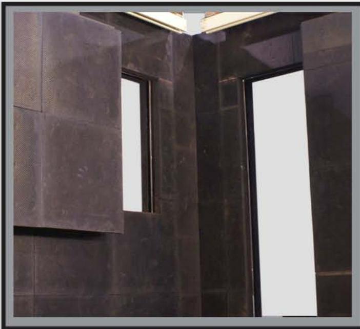
Rolling Windows and Doors.
