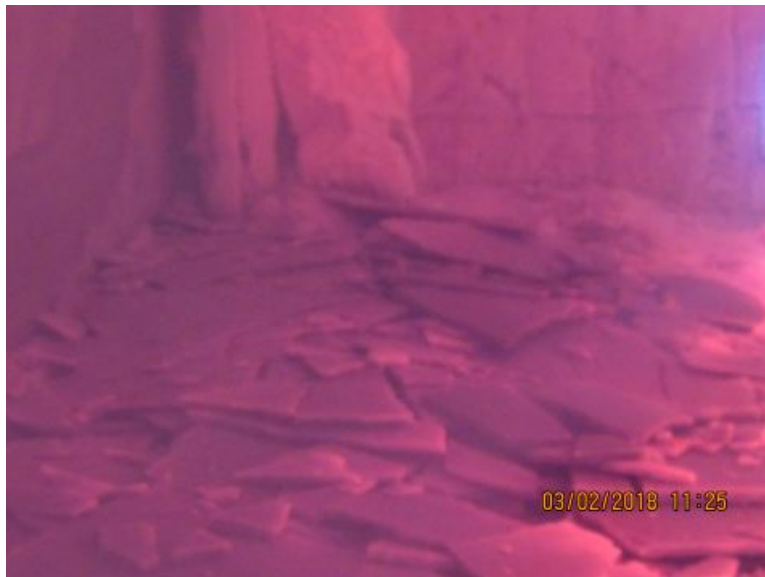
Photo No. 19 Stucco Finish Falling off Wall (Exposed Side)
