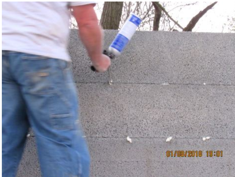
Photo No. 5 Injection of Adhesive
