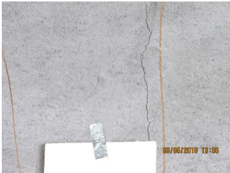
Photo No. 31 Centerline Crack Develops
