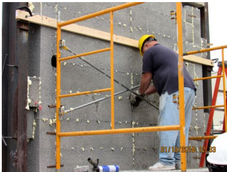
Photo No. 7 Plugging of Holes after Concrete Fill
