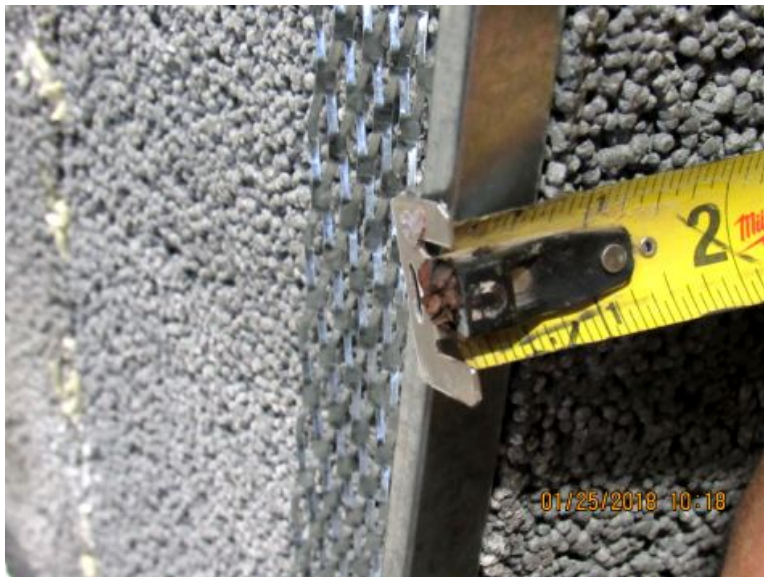
Photo No. 13 Measurement of Casing on Perimeter of Wall
