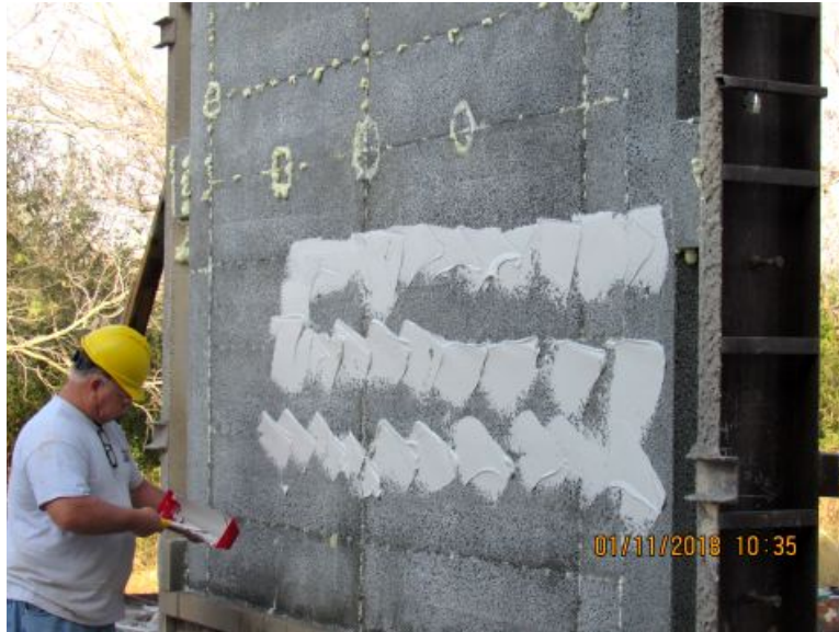
Photo No. 8 Prepping for Installation of Gypsum Board
