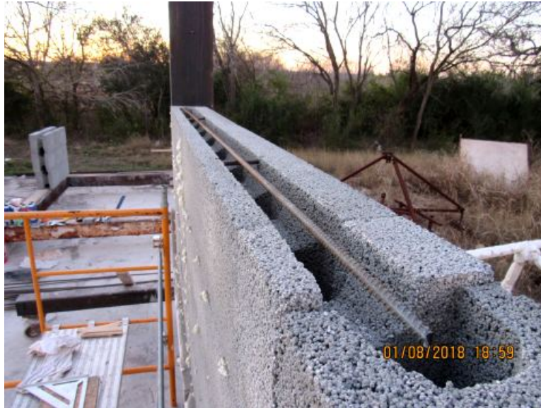
Photo No. 4 Installation of Re-bar
