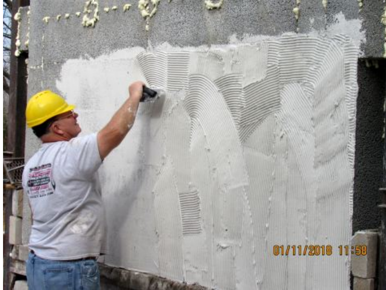
Photo No. 10 Troweling of Joint Compound
