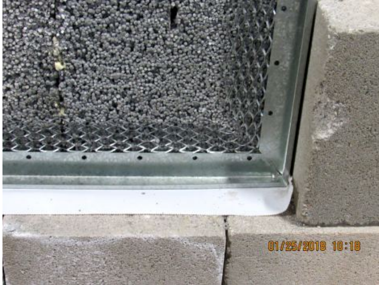
Photo No. 12 Installation of 3/4 in. Casing for Stucco
