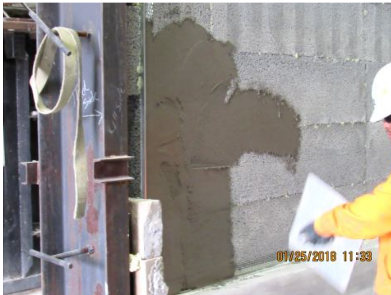
Photo No. 15 Application of Stucco
