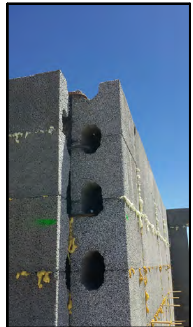
Photo 7.10 Exterior Corner, 10" Asymmetric ICCF
