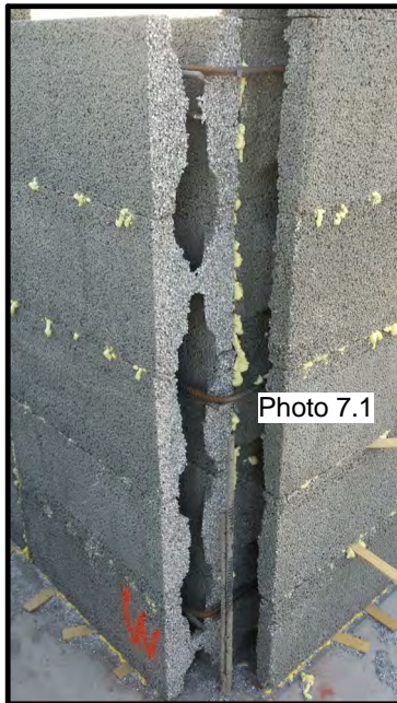
Photo 7.6a Tack gluing (every 12") of the first course.
