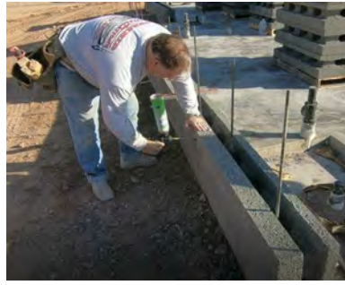
Photo 7.6b Tack gluing, both sides.
