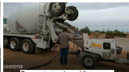
Concrete truck and line pump
