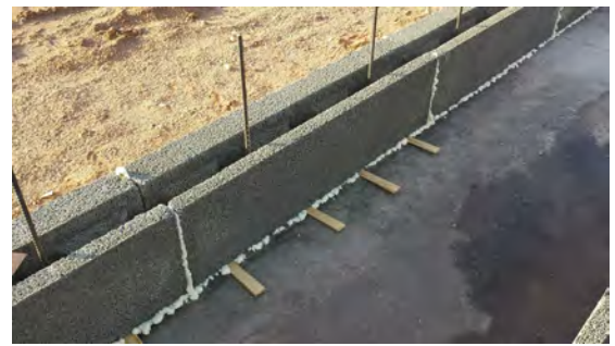
Photo 7.6c Plumb and level and polyurethane foam adhesive in place. Take great care not to move the block when tacking block in place. 15 to 20 minutes later, when the tack gluing dries, you can "super glue" (glue every 3-4") the block.
