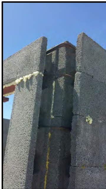
Photo 7.9 Interior Corner, 10" Asymmetric ICCF
