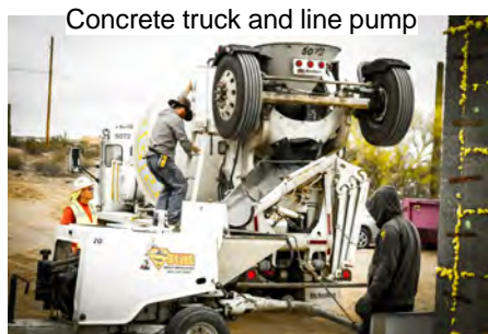
Concrete truck and line pump
