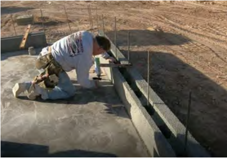
Photo 7.6a Tack gluing (every 12") of the first course.
