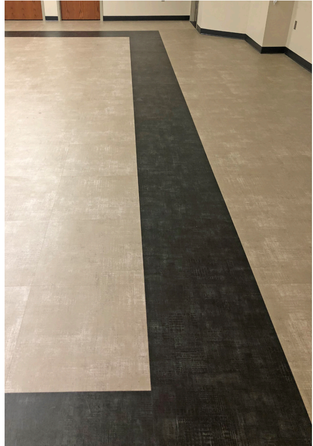
After treatment, scuffs were gone and the appearance of most scratches eliminated. There were deeper scratches that we attempted to repair with the restoration pad by hand. We were not successful and suggested replacing these tiles with attic stock.
