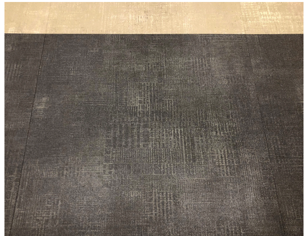
Same tiles after full treatment. Some of the deeper scratches were not removed by this more tempered approach to refurbishment in which case it was recommended to replace those tiles with attic stock and applying Vinyl Seal.
