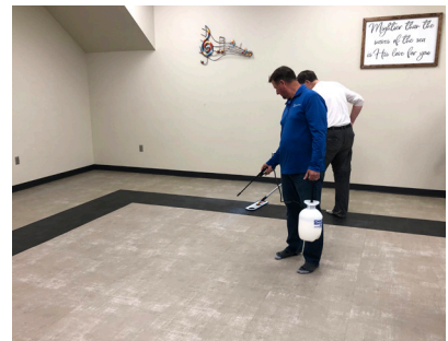
Applying the Vinyl Seal.
