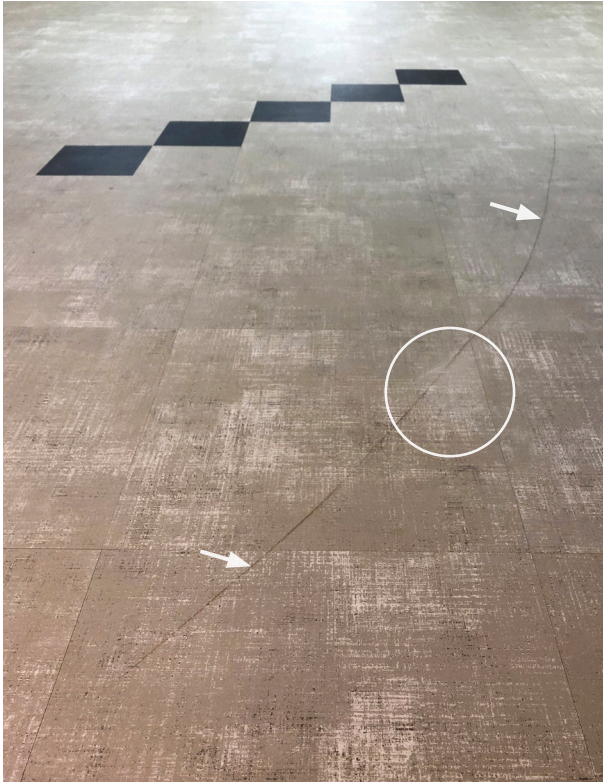
Top of entry lobby with very long arcing dark scuff. Attempts by the school to remove the mark using an abrasive sponge scrub pad resulted in a dulled-out spot (circled).
