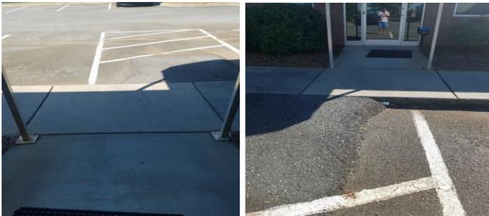
For example, a company recently bought a building for their operation. With all the fixing up, remodeling, and operations, they failed to recognize that the handicap ramp that had been installed by the previous occupant did not align with the front door. It wasn’t until an employee left one day and stepped off the curb and onto the ramp and almost fell that it came to their attention. In some organizations, they would simply tell people to be more careful and watch where they
