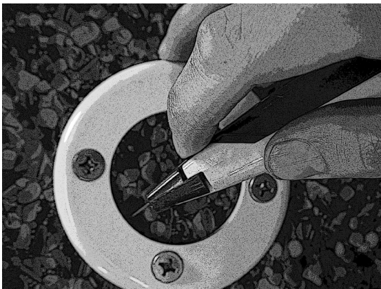
Trim liner from return opening.
