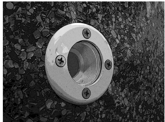
Return faceplate installed.
